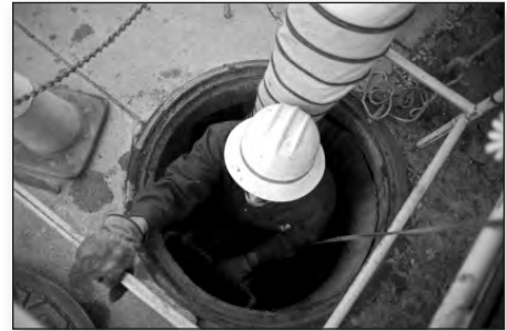
Sewer workers regularly work in confined spaces
